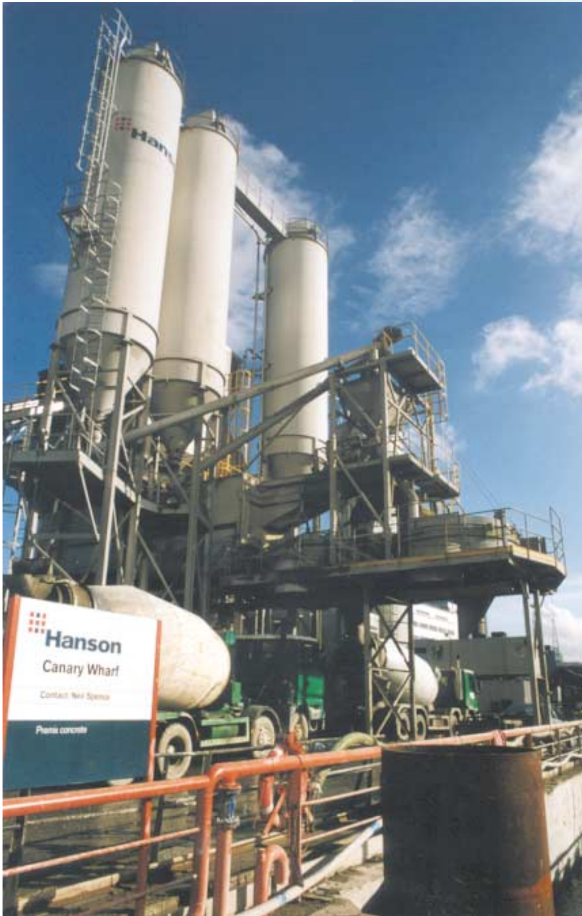
Modern ready-mixed concrete plant – rmc is made in factories under closely controlled conditions.
