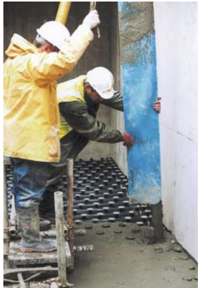
Self-compacting concrete – for difficult placing conditions or where high-quality surface finishes are required.
