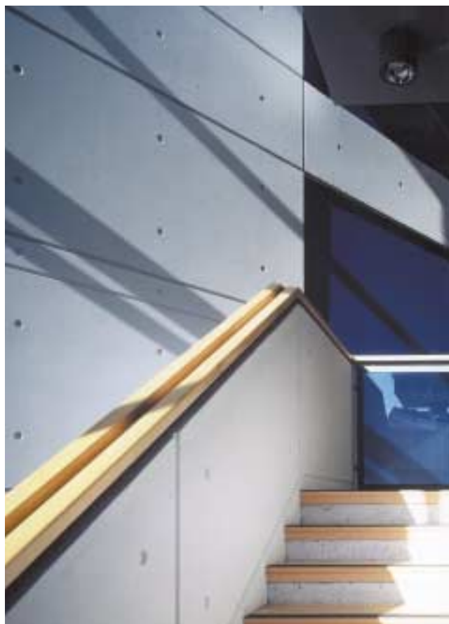
High-quality, in-situ concrete finishes at the European Institute of Health and Medical Sciences, Guildford.
