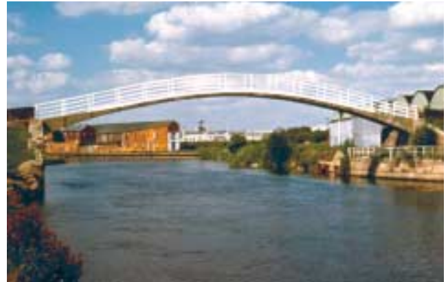
Reinforced concrete footbridge, Newark, 1915. Concrete – the material for extreme weather conditions.
