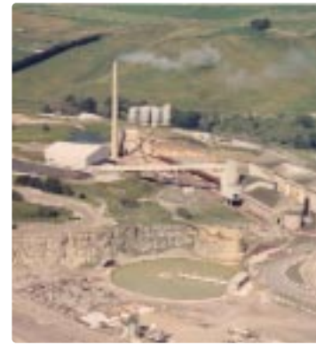
Figure 3: Imperial Chemical Industries' cement works at Tunstead, constructed 1968.
